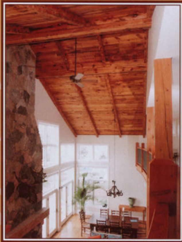
Ceiling Planed Barking Board and Hand Hewn Beam
